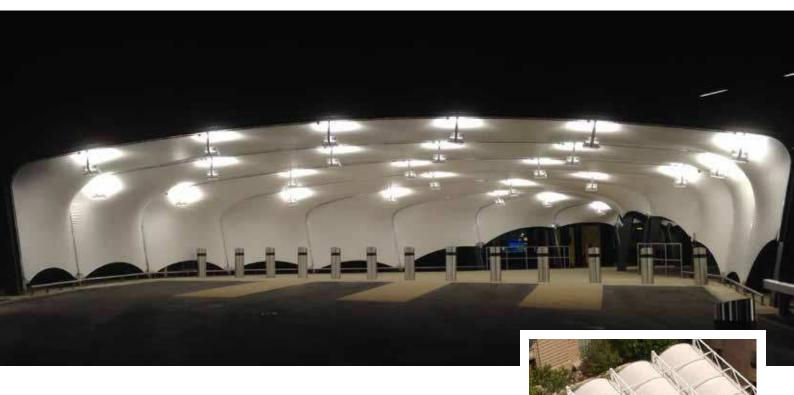
The Barrel Vault design is a symmetrical curved tensile fabric canopy which is linear in plan. It offers a simple design with a large clear span and a choice of widths, and lengths as required. As you can see from the details in the table below, we can use any of a number of architectural fabrics to create a Barrel Vault canopy including transparent ETFE to suit your requirements. All of which will have a design life of 20+ years.
