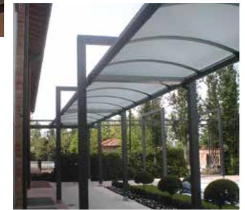
This classic mono-pitch type structure is very versatile in its sizing and use of materials. Once the basic frame is constructed it can be clad using the unique TEXO® fabric panel system which can carry any one of a number of architectural fabrics including transparent ETFE. Please take a look at our glass replacement and lean to canopy pages for further information on this revolutionary system.
