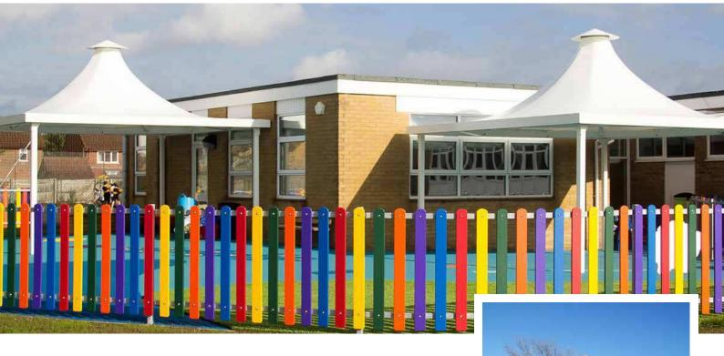
The Pavilion is a conic shaped tensile structure with a square footprint fully wind rated and snow loaded to British Standards. Its variable corner columns leave an uninterrupted space underneath the canopy that can be used for many applications such as shaded playground shelters, entrance canopies, restaurant canopies, etc. The design also benefits from a vented head ring.
